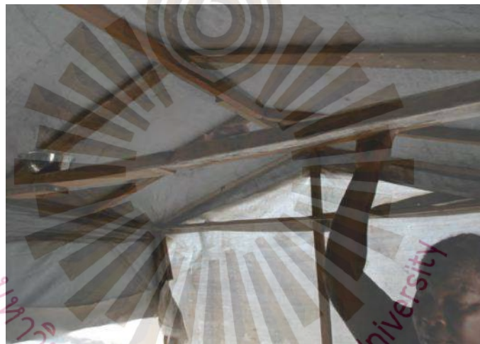
Figure 3.2 Shelter frame built with sloped roof as per suggestion
