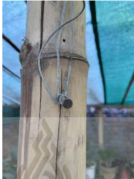
Figure 3.10 Additional methods of secure sheets to the frame
