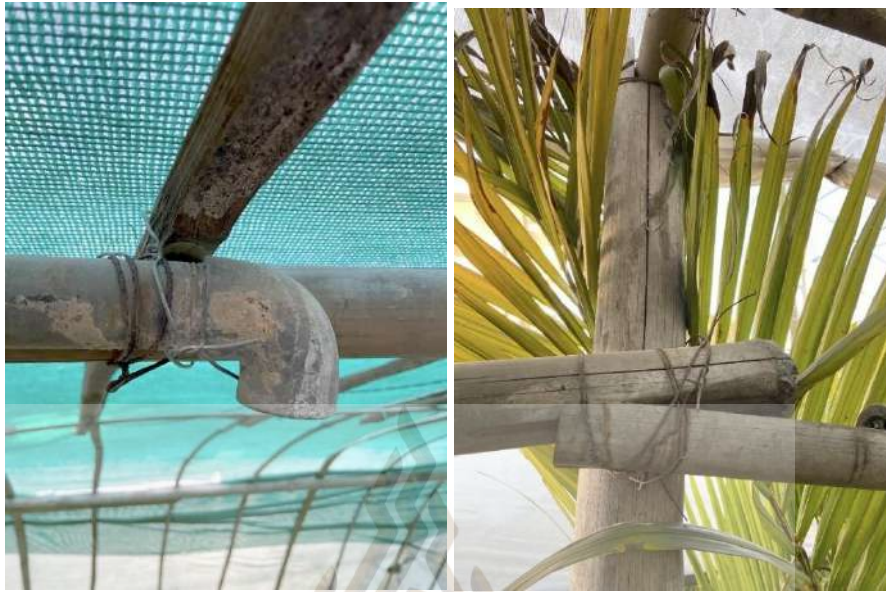
Figure 3.7 tying of two shorter materials to make longer frame
