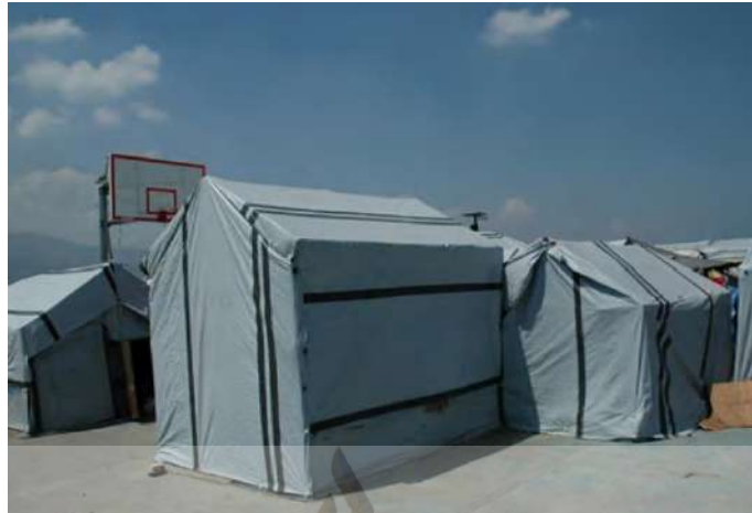
Figure 3.3 Adequate sheet installations to prevent wear and tear
