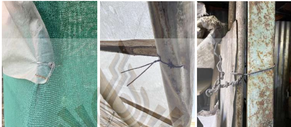
Figure 3.9 Use of wire to secure materials to frame
