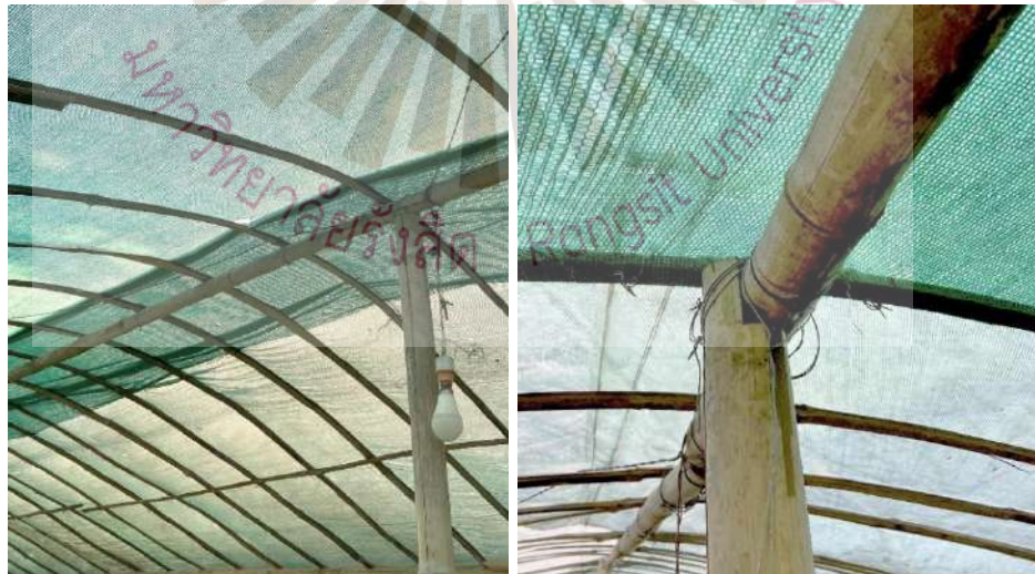
Figure 3.8 Raised roof for rainwater drainage
