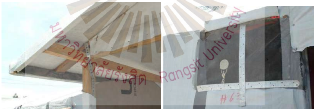
Figure 3.4 Use of hurricane straps to secure structures
