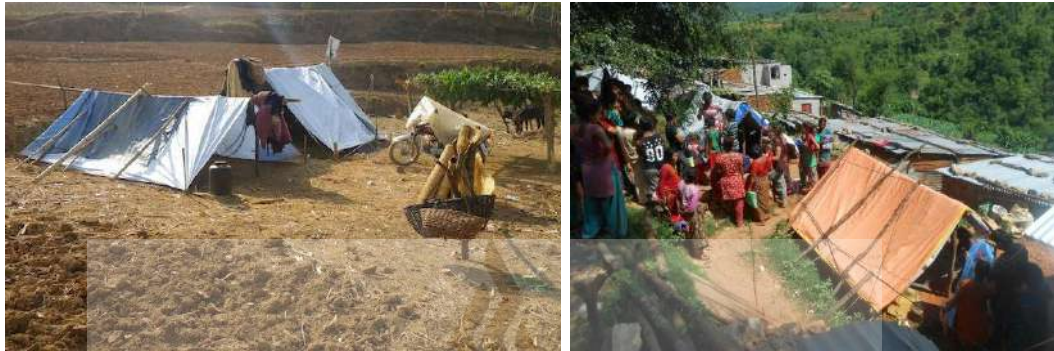
Figure 3.5 Use of logs as weights on shelters
